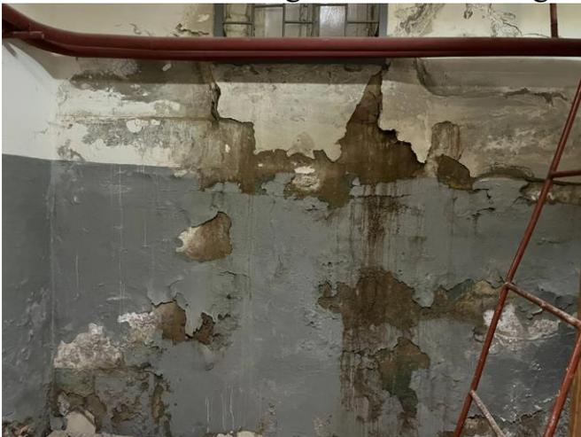
Figure 1 - Wetting of the wall structure
