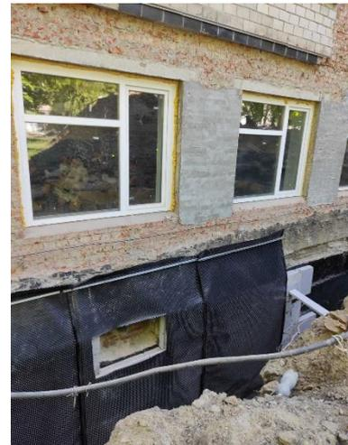
Figure 2 - Thermal insulation of the wall structure
